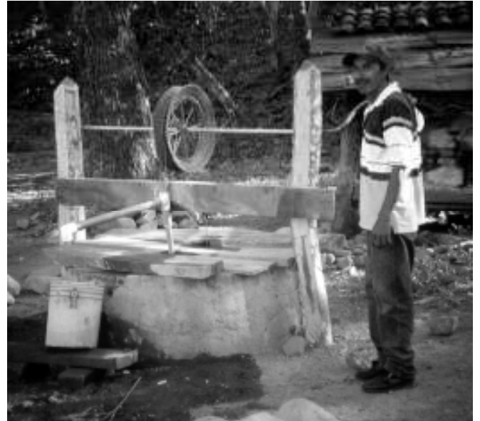
Rope pump in use at the La Poma well.
